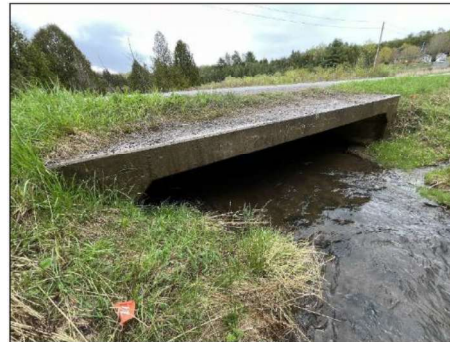
Elgar Drive Culvert – Good Condition
