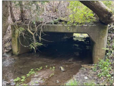
Sharp Line Culvert – Fair Condition
