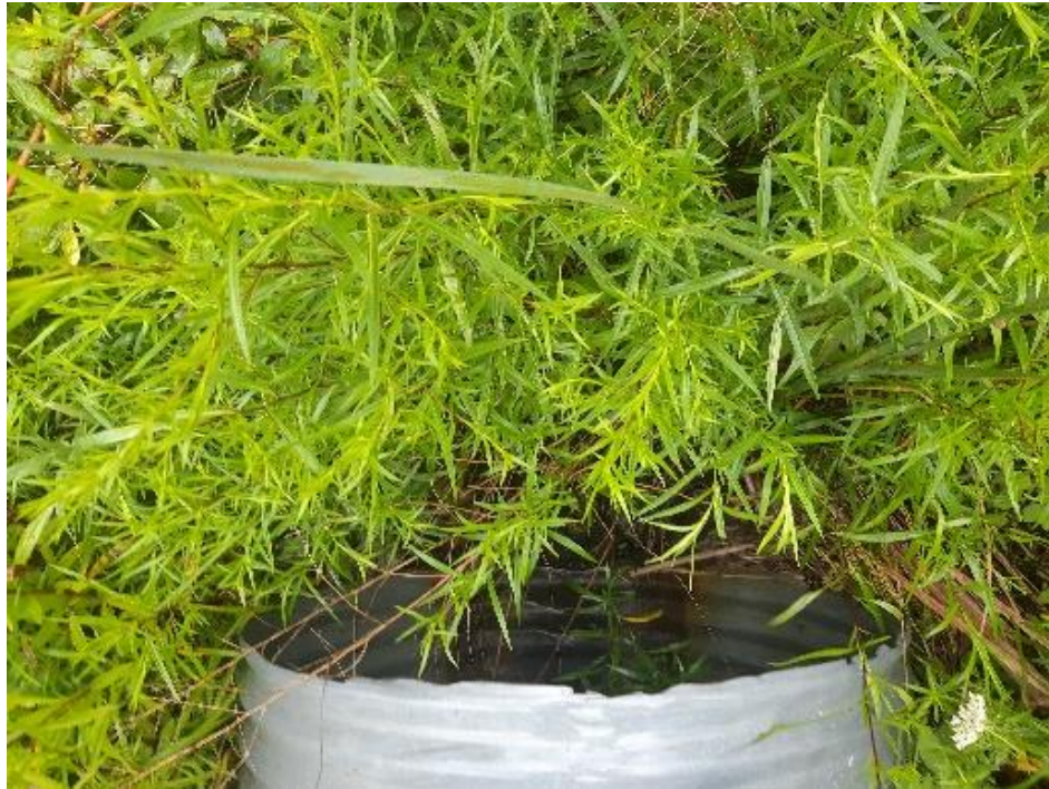
Syer Lane culvert, east of laneway, looking south
