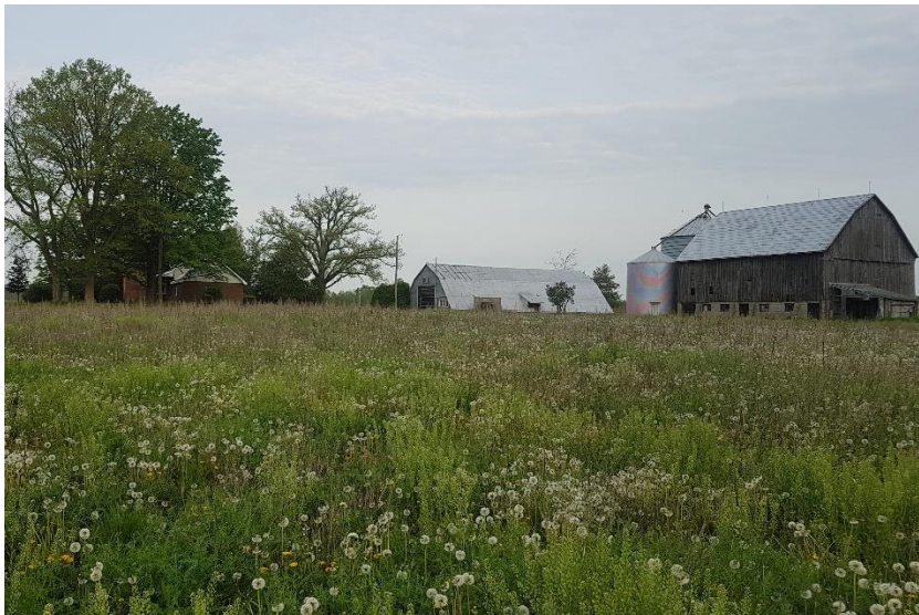
Barn structure and silo located on the northeast side of the property, looking northwest. (TJ)
