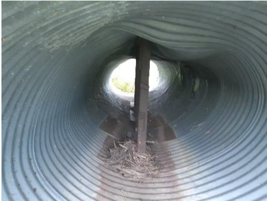
Laneway culvert interior.
