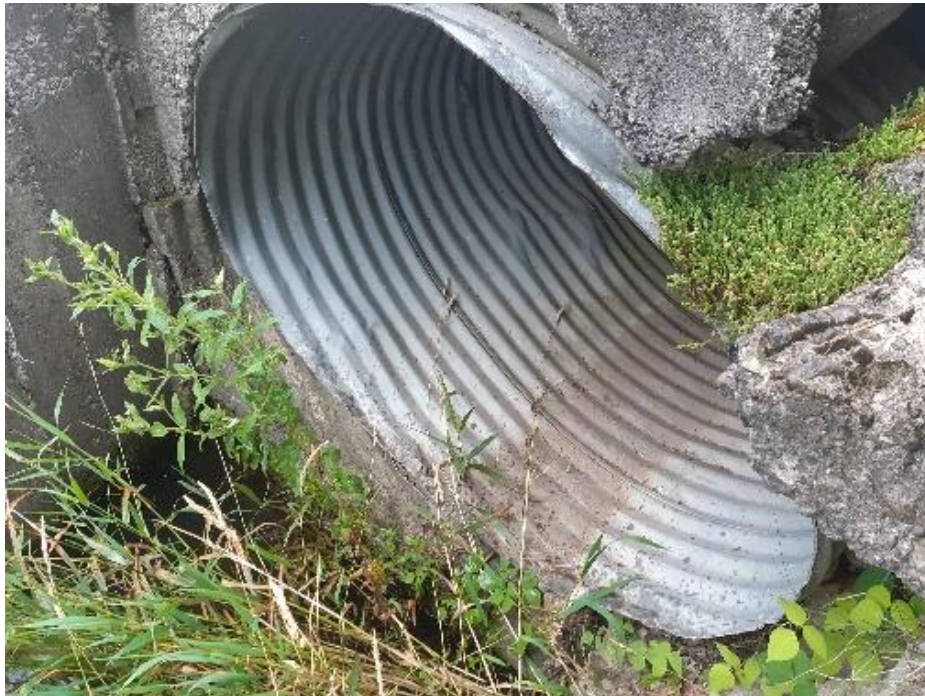
Laneway culvert, east side
