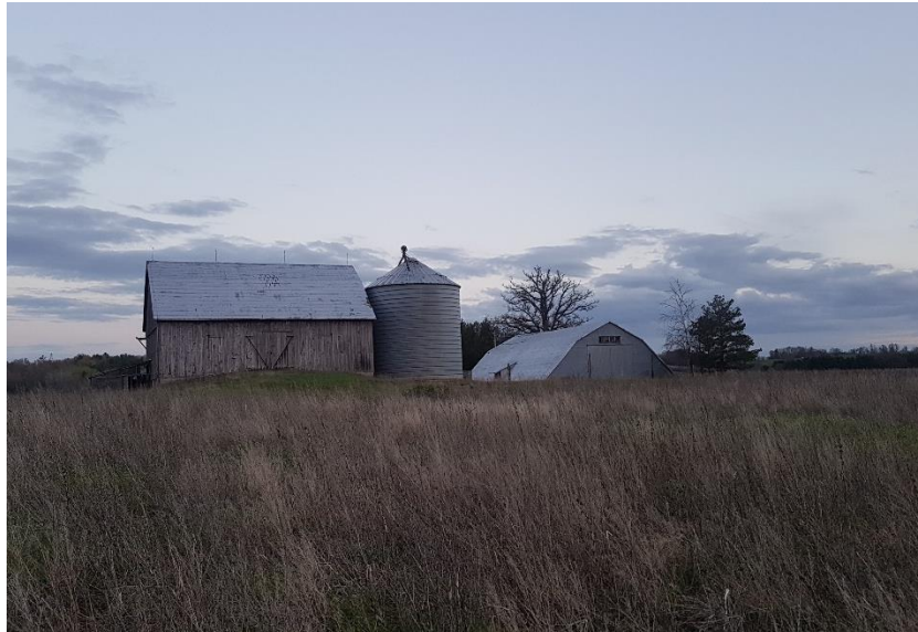
Barn structure and silo located on the northeast side of the property, looking south. (TJ)
