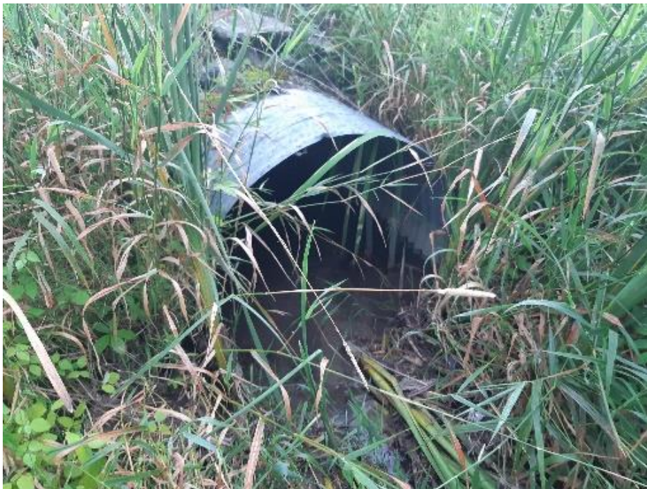
Syer Line culvert, east of laneway, looking north
