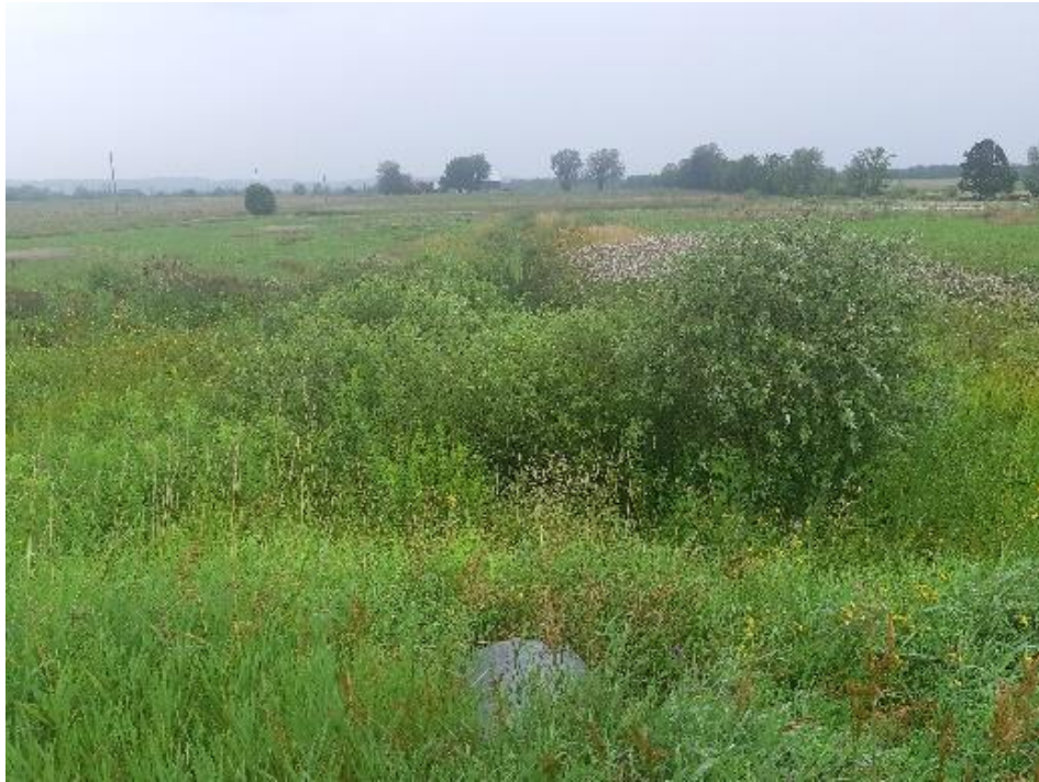
Syer Line culvert, west of laneway, looking north
