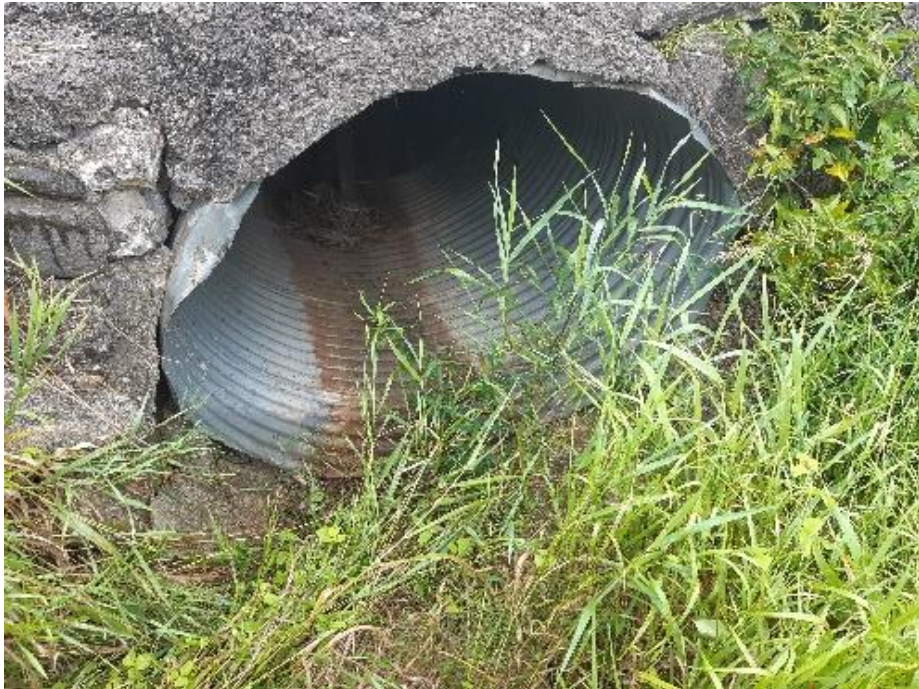
Laneway culvert, west side.
