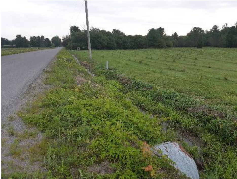
Syer Line culvert, east of laneway, looking south
