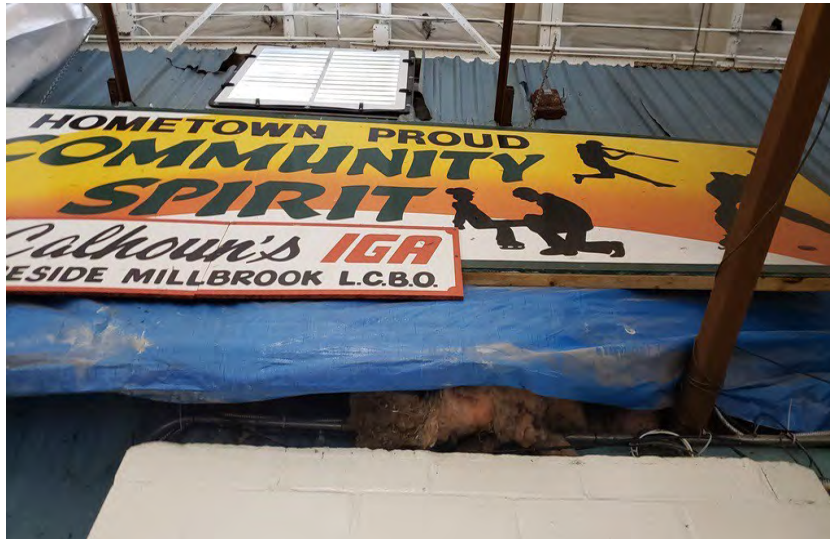
Photo 014 Metal Cladding Damage
