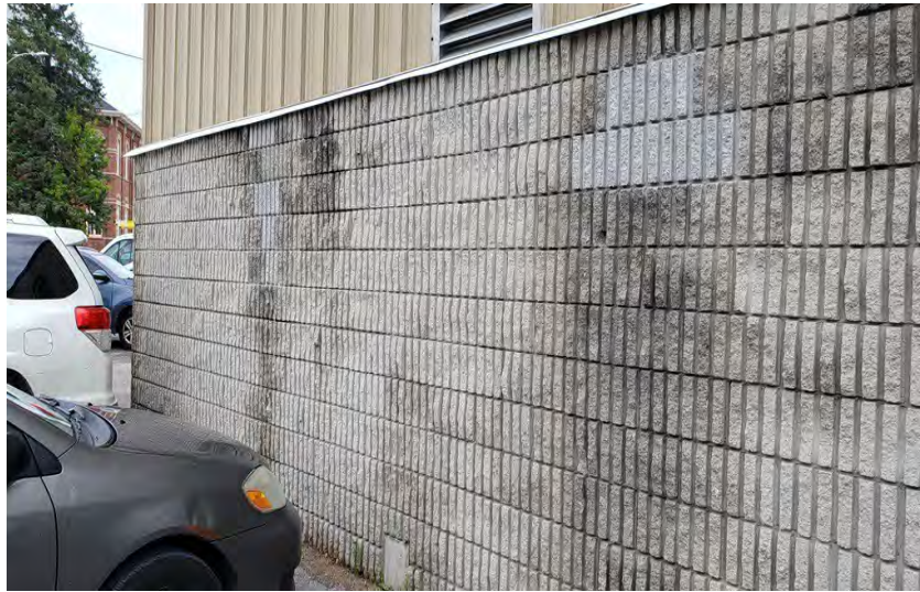
Photo 068 Architectural Precast Concrete Wall Panels
