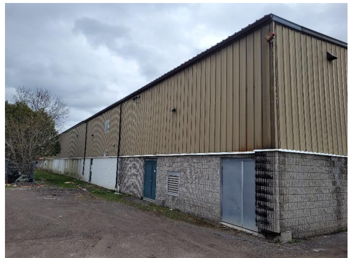
Photo 24 – Part West Elevation
