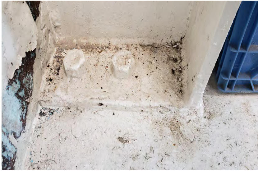
Photo 007 Pre-Eng Frame Base Connections
