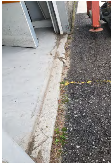
Photo 018 Apron Slab Under Garage Door
