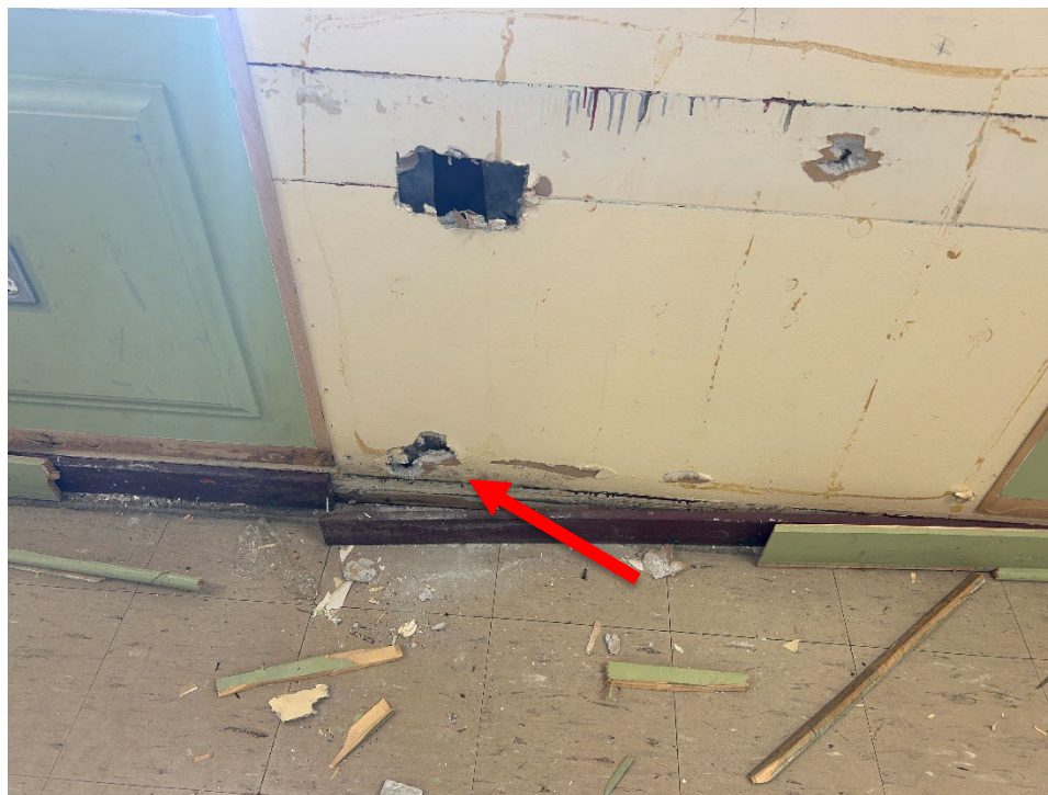
Photo 3 Mould growth on gypsum wall and wood baseboard trim in the second floor hall.
