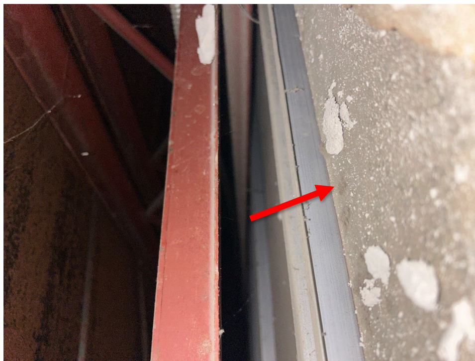
Photo 4 Mould growth on gypsum in changeroom 3.
