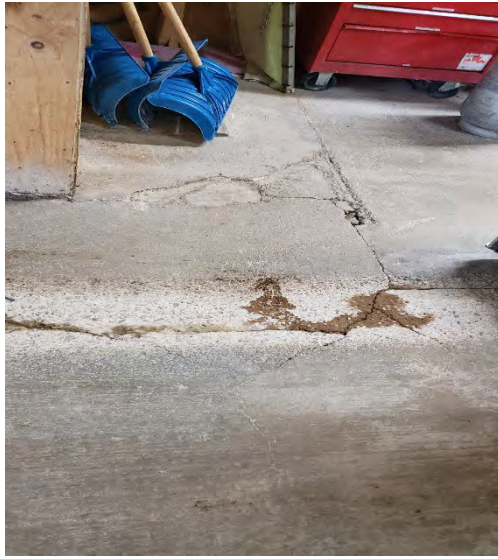
Photo 021 Cracking Starting in Resurfacing Room
