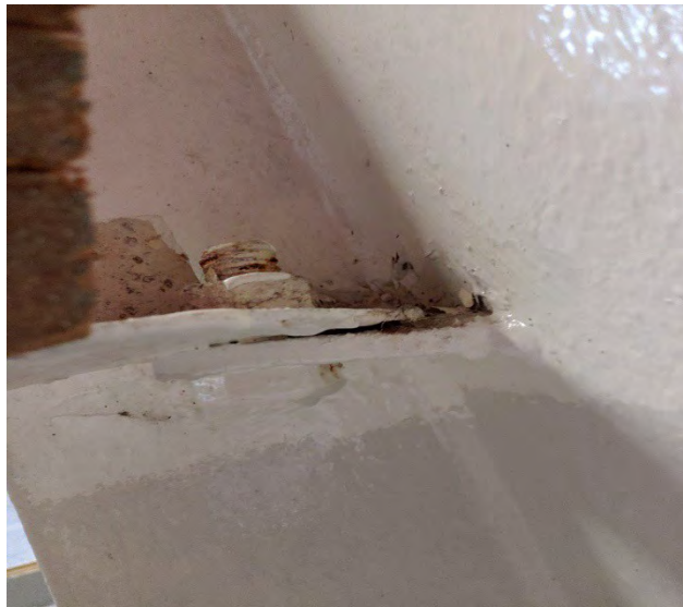
Photo 006 Rusted Bracing Connection
