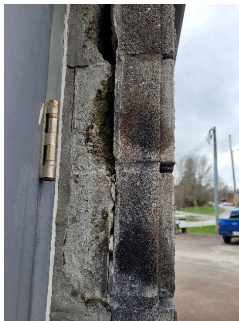
Photo 26 – Damaged Split Ribbed Block at Southwest Corner
