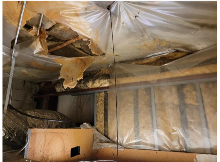
Photo 18 – Mould and Evidence of Moisture
