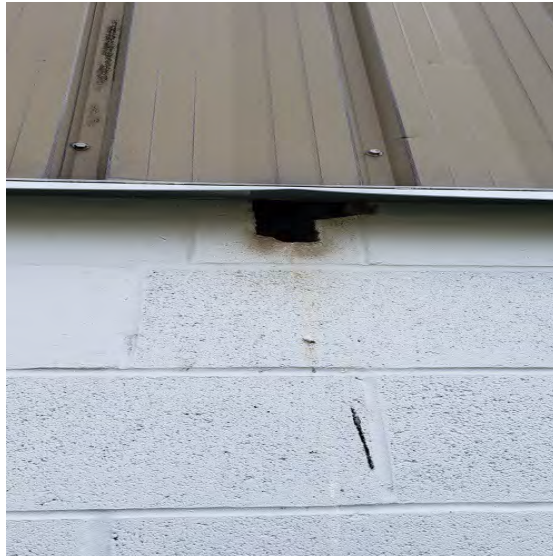
Photo 093 Hole in Masonry Block
