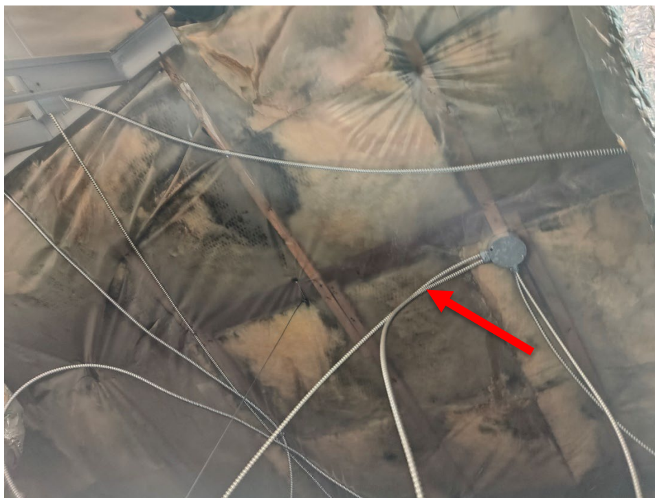
Photo 8 Mould growth on vapour barrier and fibreglass ceiling insulation.
