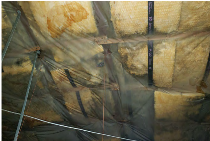
Photo 060 Moisture in Roofing System
