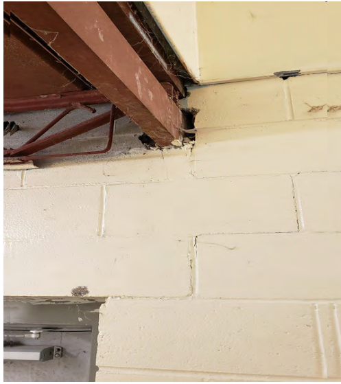
Photo 047 Localized Block Failure
