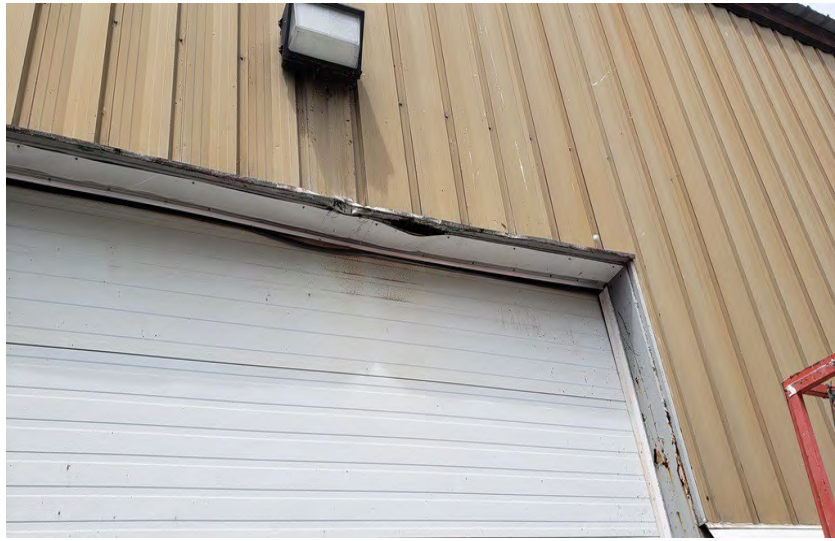
Photo 077 Damage to Garage Door Opening
