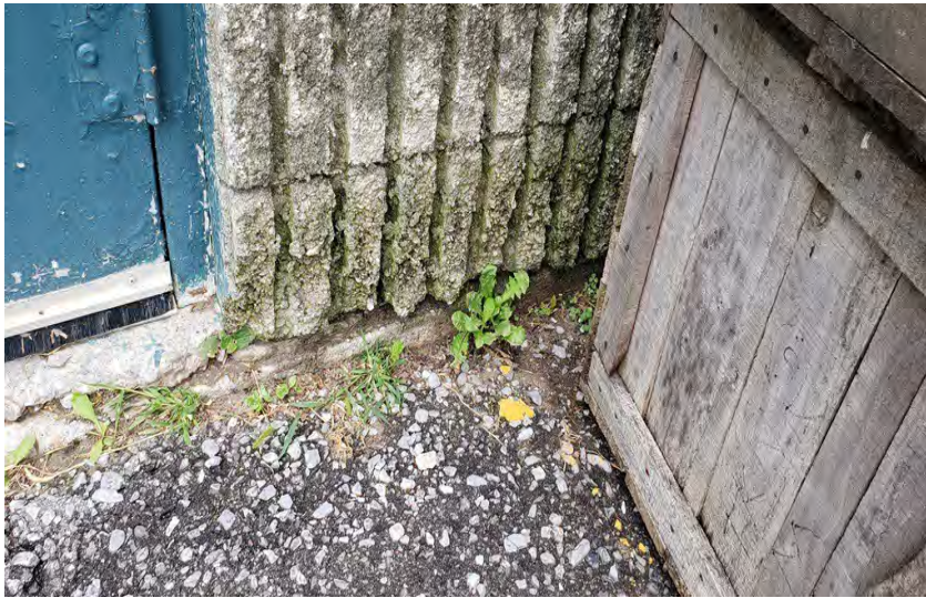
Photo 074 Deterioration of Blocks
