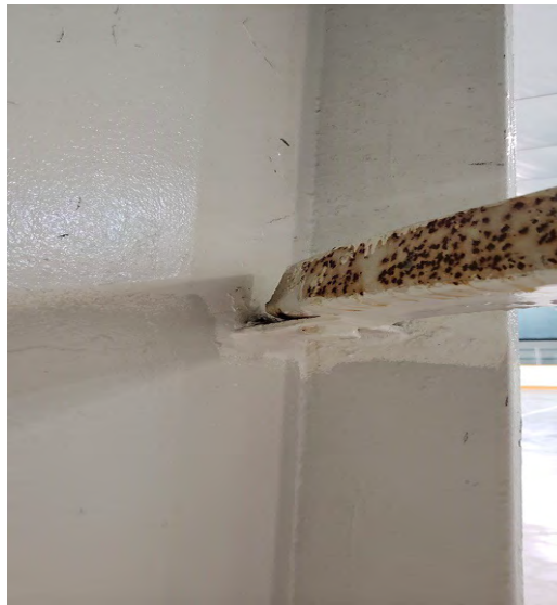
Photo 004 Rust on Frame Brace
