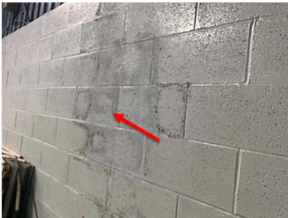
Photo 10 Mould growth concrete block wall.
