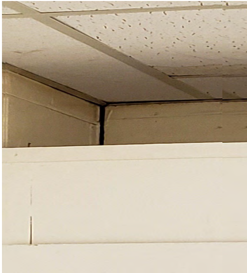
Photo 049 Wall Separation in Second-Floor Storage Room
