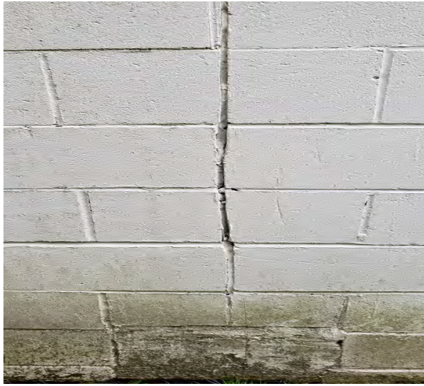
Photo 091 Damaged Wall Joint
