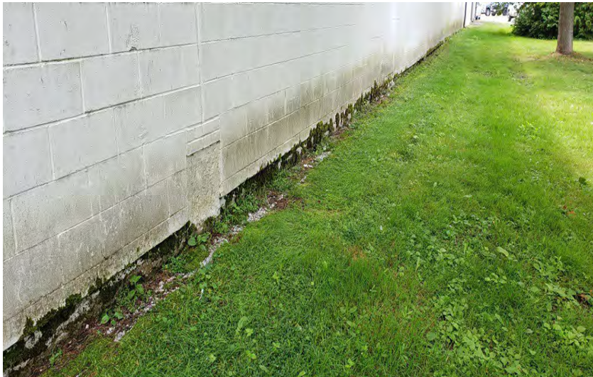
Photo 090 Mould Along West Side
