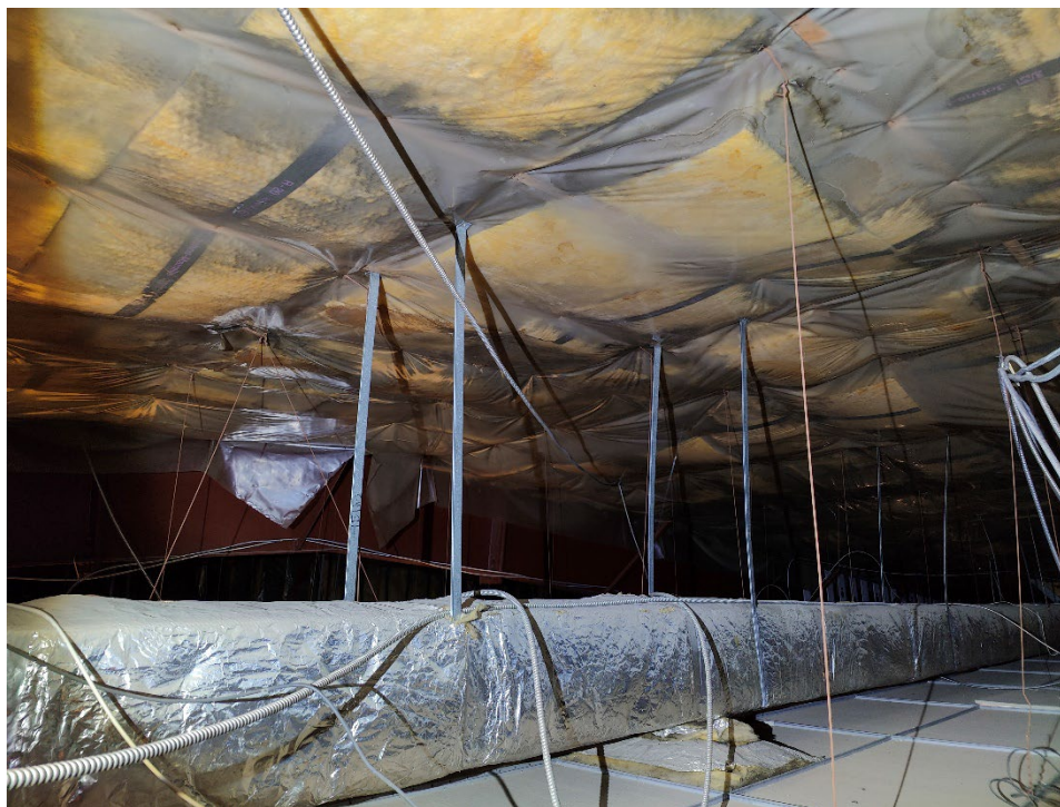
Photo 9 Mould growth vapour barrier and fiberglass insulation.
