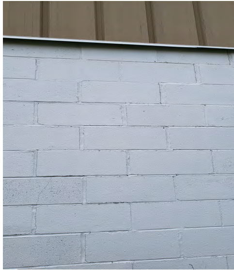
Photo 081 Step Cracking and Block Failure
