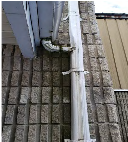
Photo 072 Damaged Eaves
