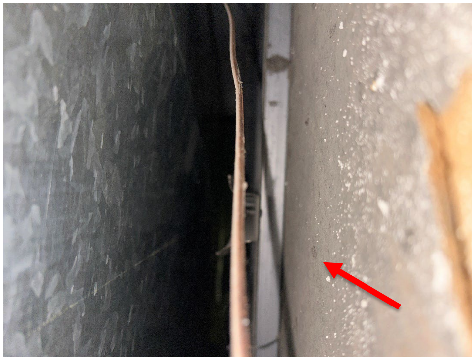
Photo 15 Mould impacted gypsum ceiling.
