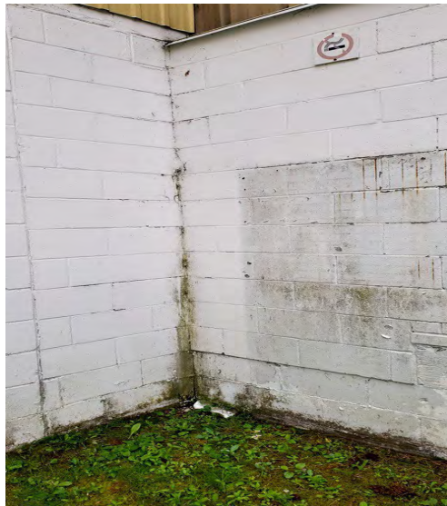
Photo 088 Mould and Moisture on Block Wal
