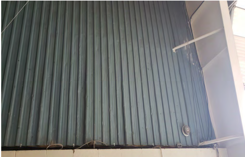
Photo 012 Localized damage to MetalCladding
