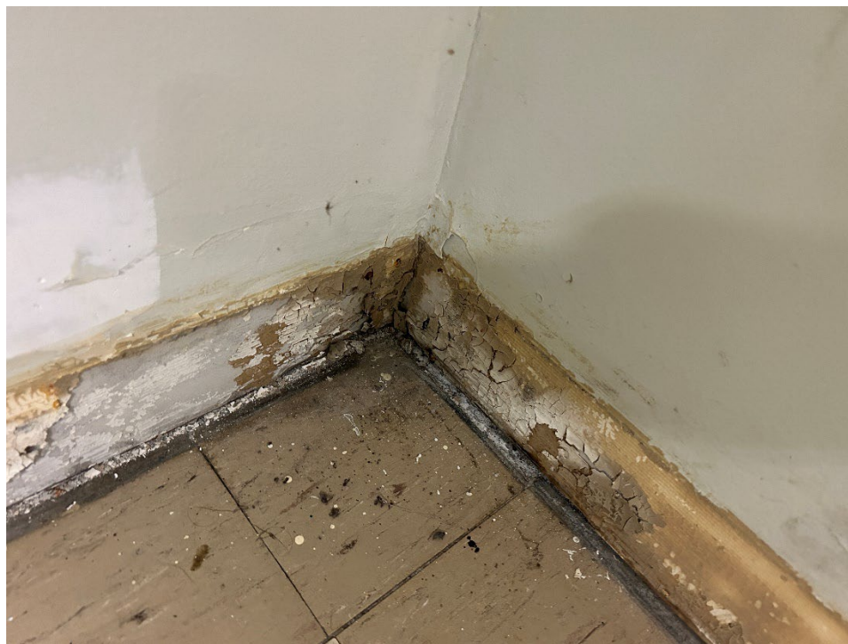
Photo 5 Mould growth on gypsum in the second-floor woman's washroom.
