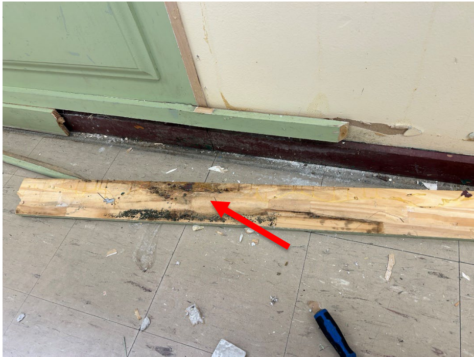
Photo 13 Mould impacted wooden baseboard.
