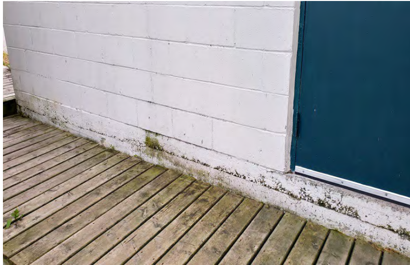
Photo 083 Honeycombing and Mould at Eastside of Ice-resurfacing Room
