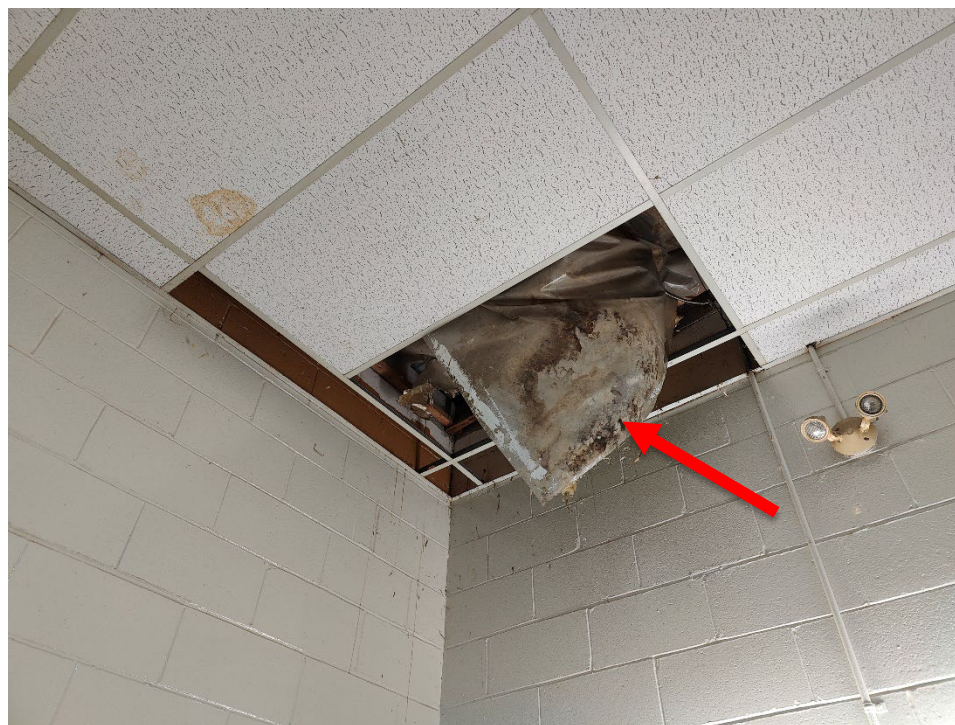
Photo 6 Mould growth on vapour barrier along with water-stained ceiling tiles.
