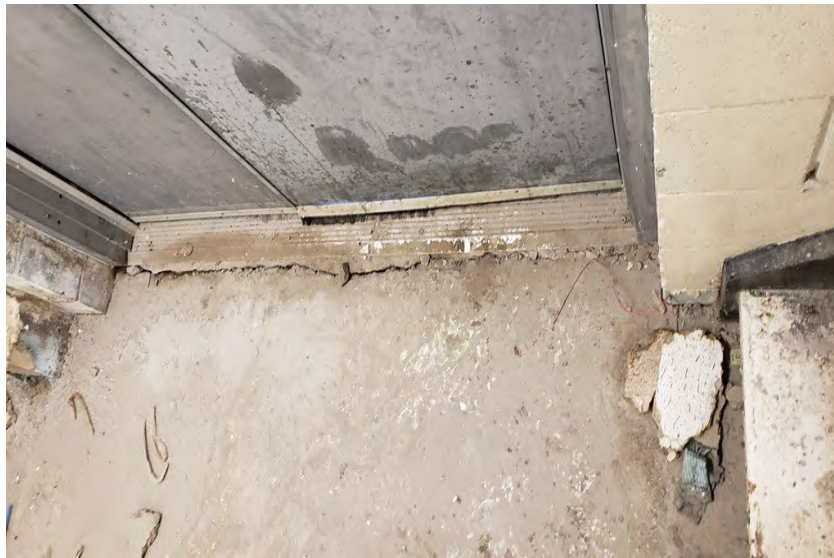
Photo 054 Slab-On-Grade Damage in West-Side Stairwell
