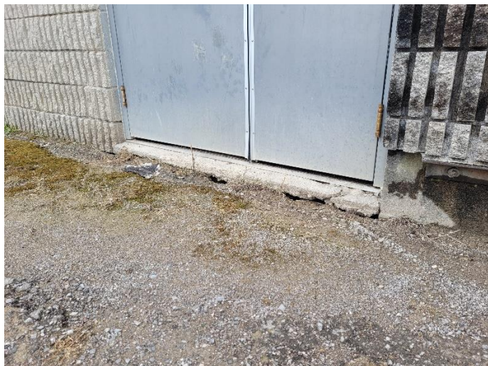
Photo 25 – Damaged Concrete Slab at Southwest Corner
