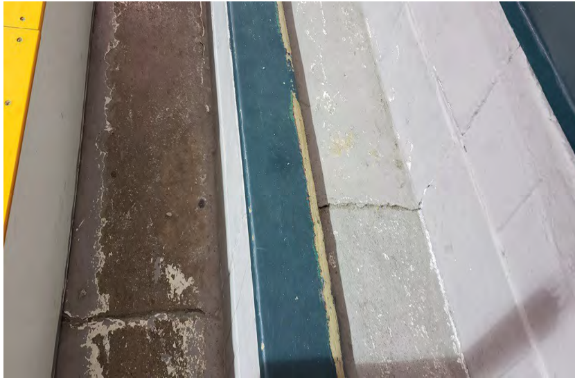
Photo 011 Bleacher Crack at Joint Location
