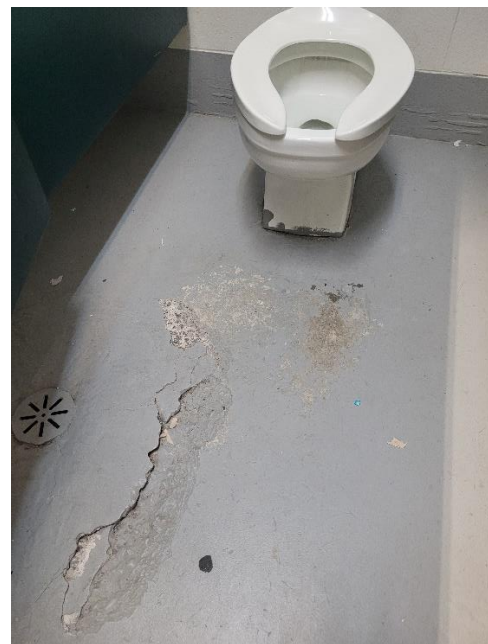
Photo 12 – Damaged Slab in Washroom
