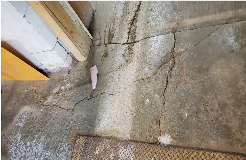
Photo 022 Extents of Resurfacing Room Cracking
