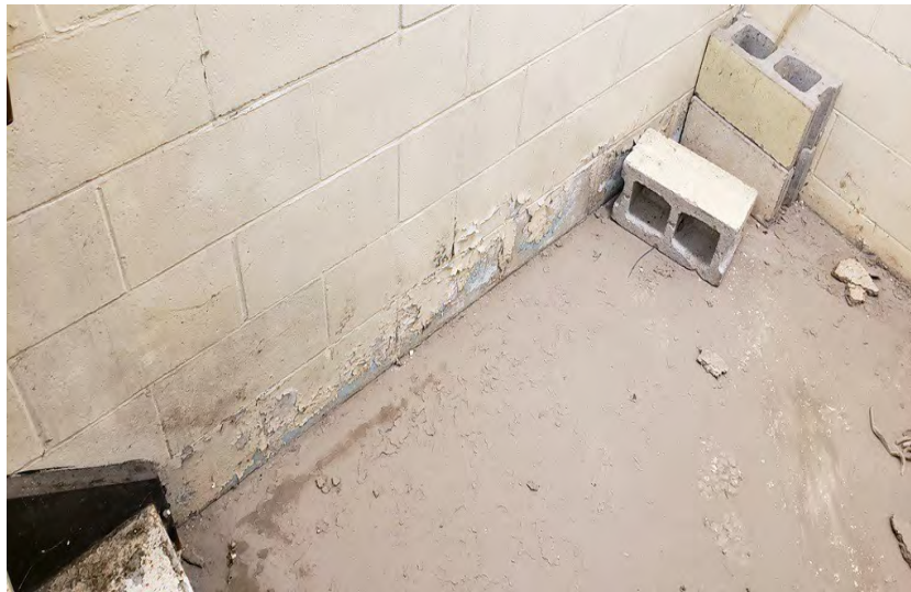
Photo 046 Paint Chipping and Moisture Damage
