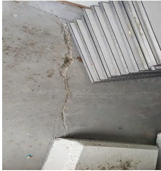
Photo 017 Cracking Outside of Compressor Room
