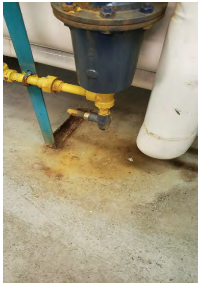
Photo 052 Concrete Staining in Compressor Room
