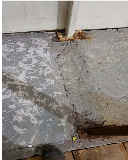
Photo 025 Crack Underneath Mechanical Equipment Stand
