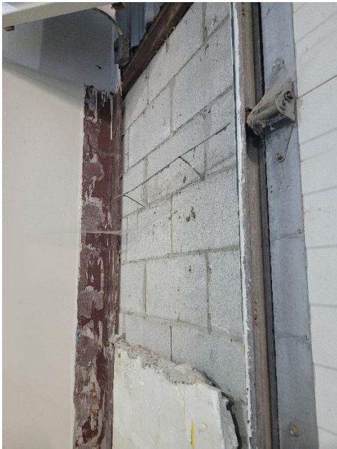
Photo 05 – Damaged Block Wall
