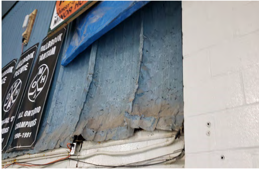
Photo 013 Significant Damage to Metal Cladding
