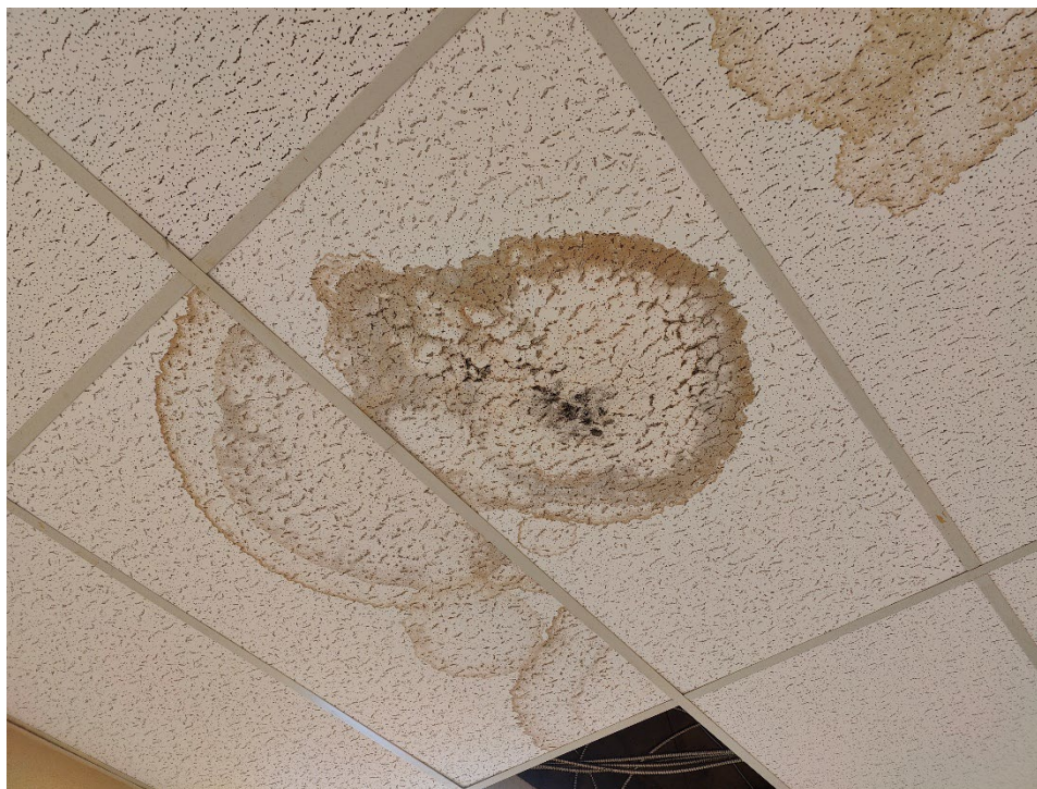
Photo 7 Mould growth on acoustic ceiling tiles.
