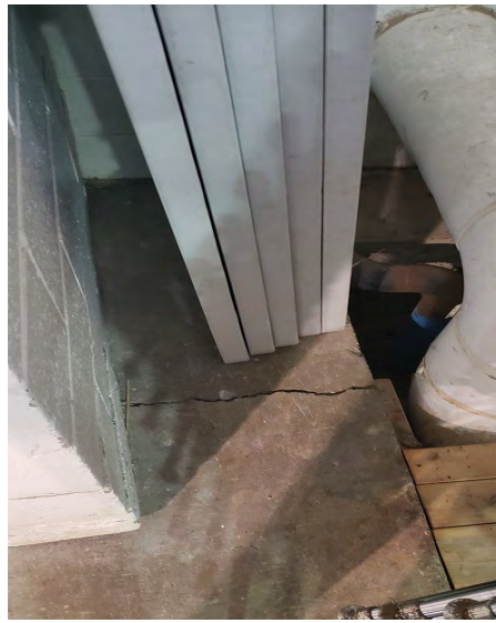
Photo 019 Major Crack in Apron Slab
