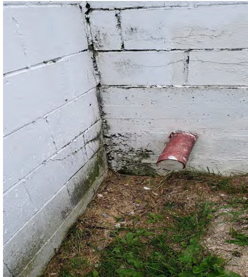
Photo 082 Honeycombing and Mould Growth
