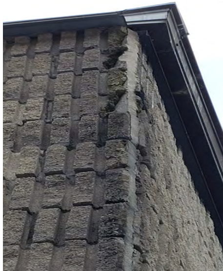
Photo 067 Localized Block Damage at South-East Corner
