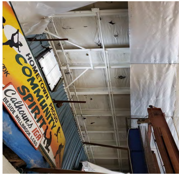
Photo 001 Hidden Roof Deck & Z-Purlins
