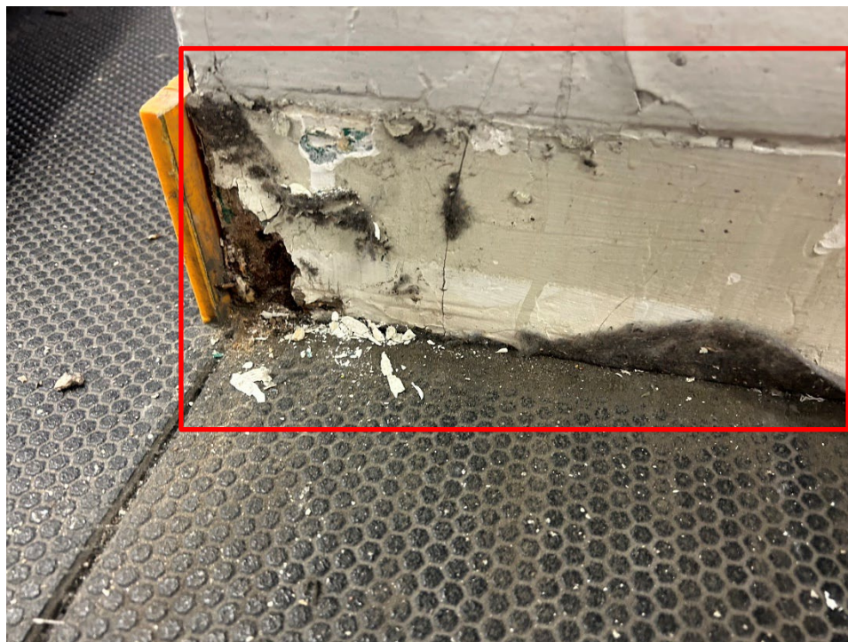
Photo 2 Mould growth on gypsum in the lobby.
