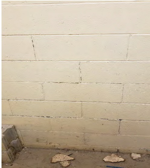
Photo 031 Minor Step Cracking in West-Side Stairwell
