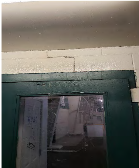
Photo 030 Step Cracking in Lobby
