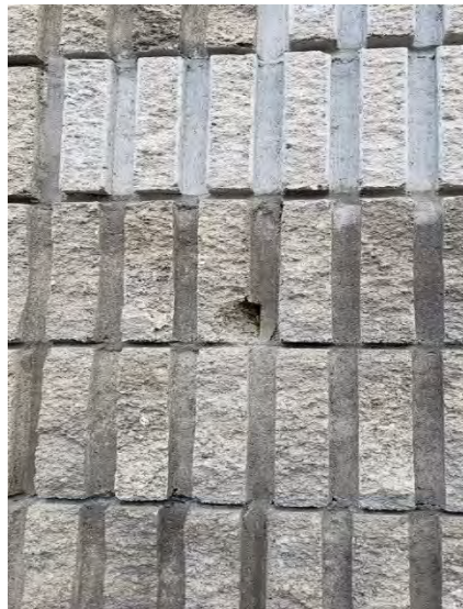
Photo 066 Localized Brick Damage
