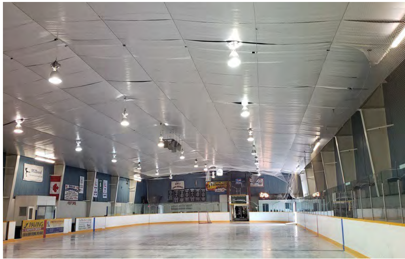
Photo 002 Roof Deck Insulation covering Pre-Engineered Frames
