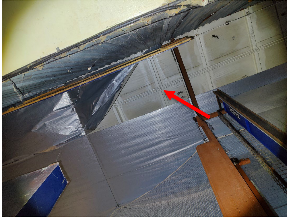
Photo 11 Mould impacted fibreglass insulation.
