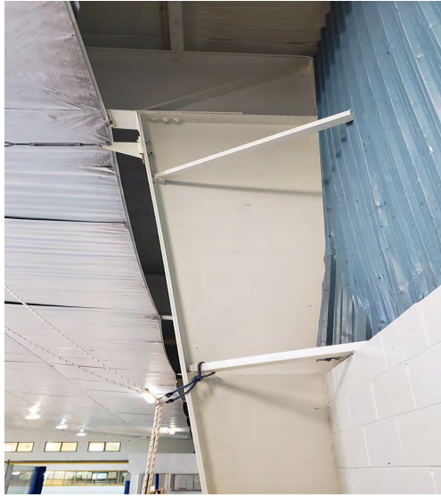
Photo 003 Pre-Engineered Frame
