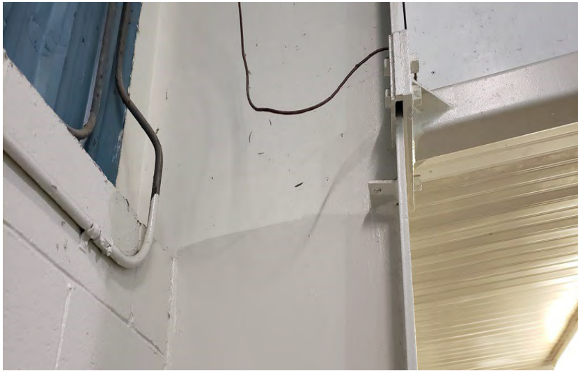
Photo 008 Missing Brace at Southmost Frame
