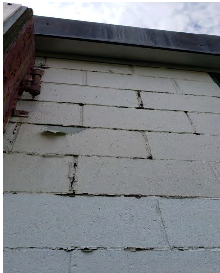
Photo 080 Step Cracking and Paint Peeling
