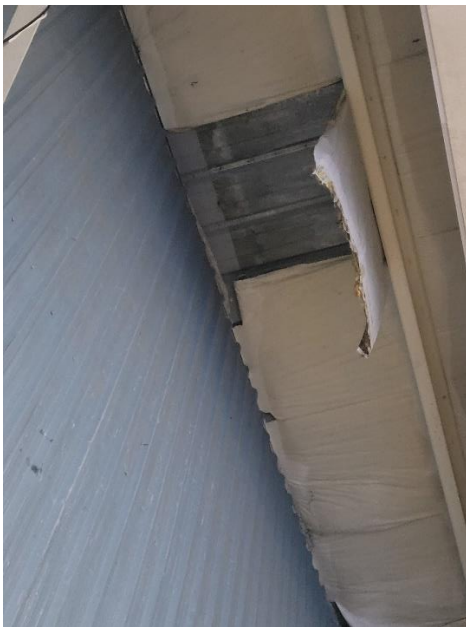
Photo 03 – Damaged Roof Insulation
