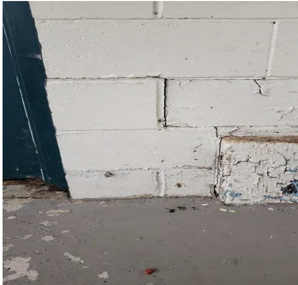
Photo 039 Step Cracking and Damage to West-Side Exit
