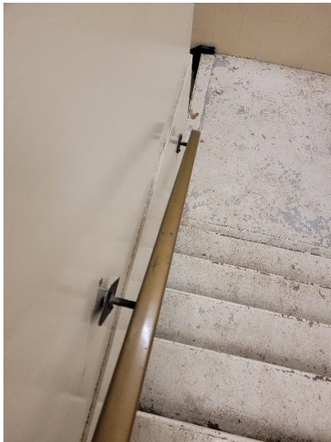
Photo 19 – Damaged Rail
