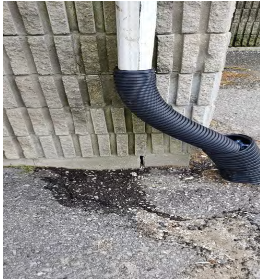
Photo 071 Gap in Foundation Wall
