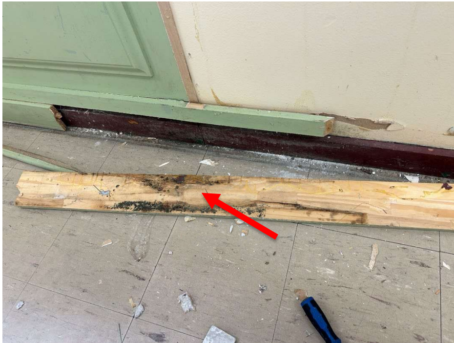
Photo 13 Mould impacted wooden baseboard.
