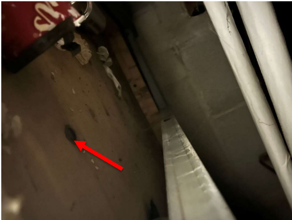
Photo 14 Mould impacted gypsum ceiling.
