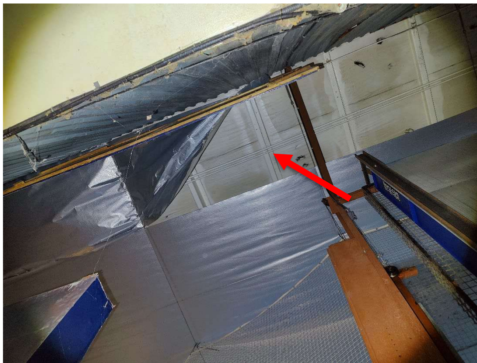
Photo 11 Mould impacted fibreglass insulation.
