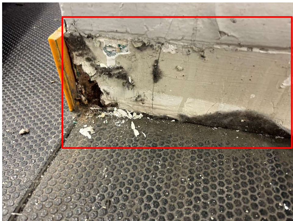
Photo 2 Mould growth on gypsum in the lobby.
