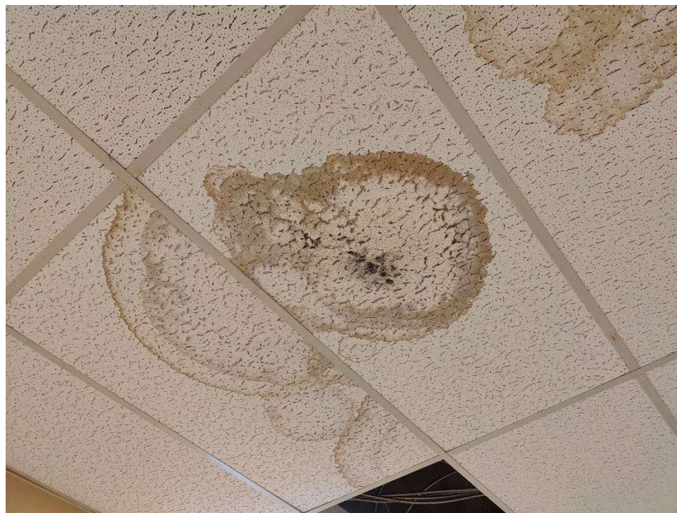
Photo 7 Mould growth on acoustic ceiling tiles.
