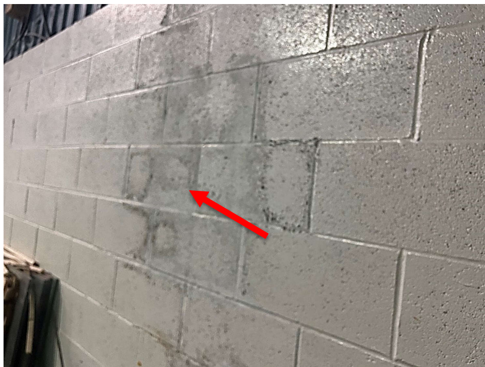
Photo 10 Mould growth concrete block wall.
