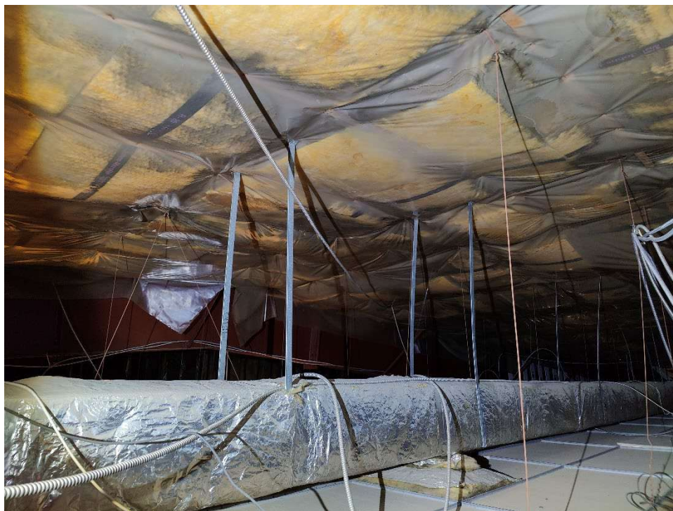
Photo 9 Mould growth vapour barrier and fiberglass insulation.
