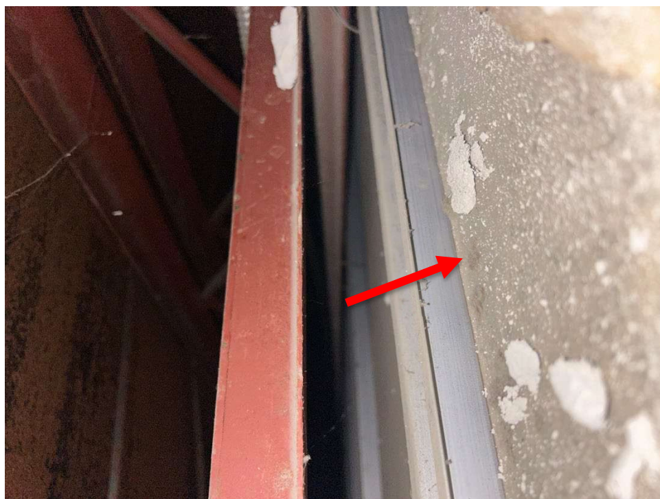
Photo 4 Mould growth on gypsum in changeroom 3.
