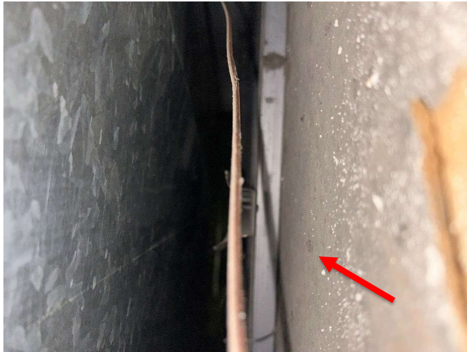
Photo 15 Mould impacted gypsum ceiling.
