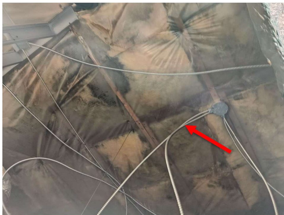
Photo 8 Mould growth on vapour barrier and fibreglass ceiling insulation.
