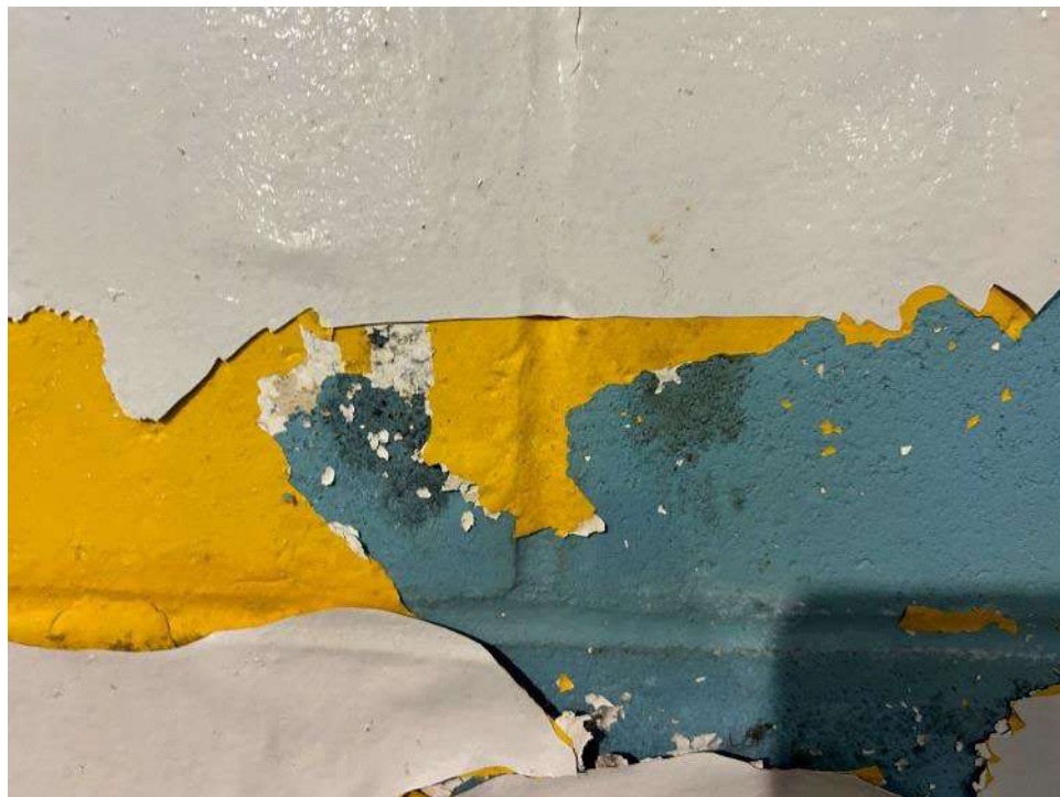
Photo 1 Mould growth on concrete in the main arena area.
