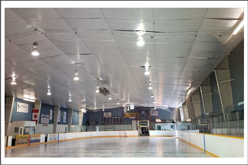
Photo 002 Roof Deck Insulation covering Pre-Engineered Frames
