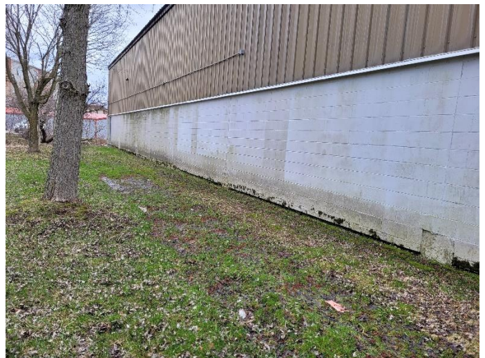
Photo 28 – Part West Elevation
