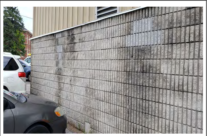
Photo 068 Architectural Precast Concrete Wall Panels
