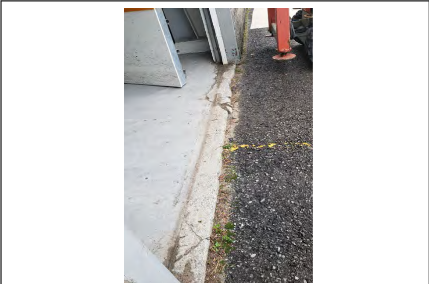
Photo 018 Apron Slab Under Garage Door
