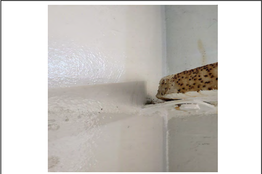
Photo 005 Bent Connection
