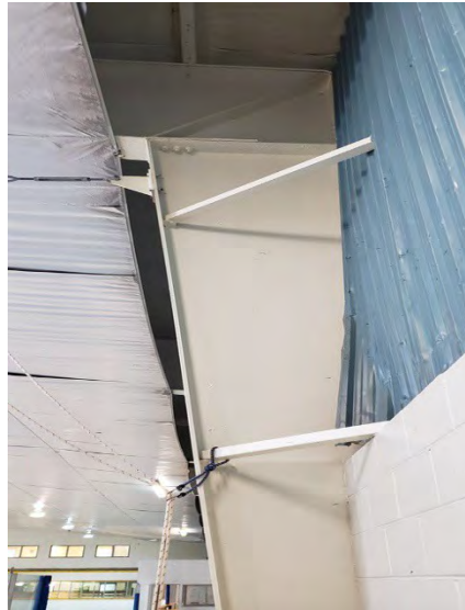
Photo 015 Metal Cladding Along West Side
