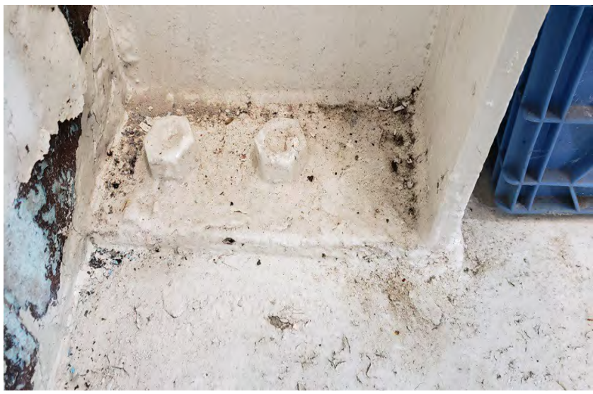
Photo 007 Pre-Eng Frame Base Connections
