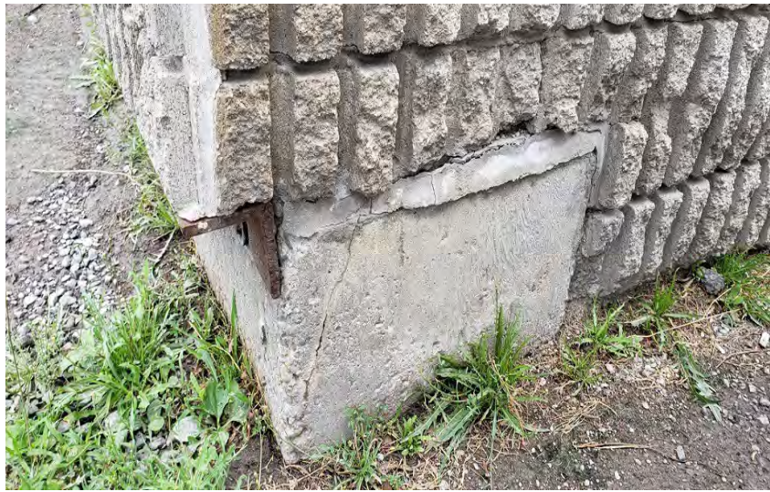
Photo 063 South-West Corner Foundation
