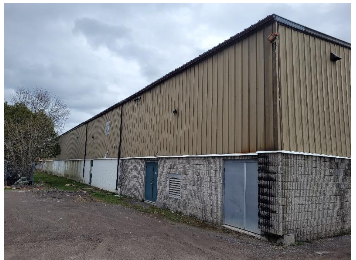
Photo 24 – Part West Elevation
