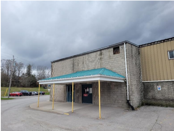
Photo 29 – Arena Entrance on East Elevation
