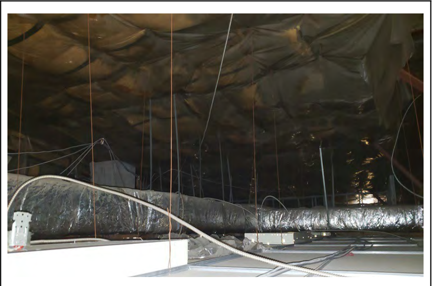
Photo 058 Insulation and Plastic Covering
