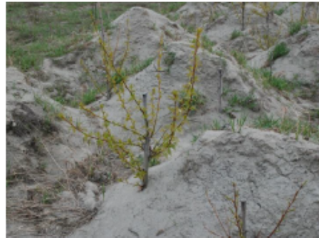
Photograph 5 (left) and 6 (right). Live staking in the rough and loose soils of this tailings pond is easy and allows the cuttings to grow rapidly (right, start of 2 nd year growth for cuttings)
