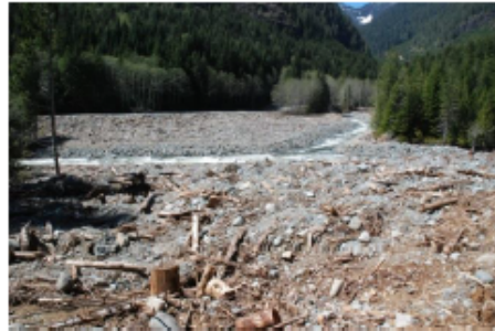
Photograph 3 (left) and 4 (right). Forest access roads and other small areas can be treated using the rough and loose technique (left) as well as areas with coarse substrates (right) such as this old dam site with alluvial boulders, cobbles and gravels.
