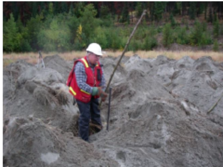
Photograph 5 (left) and 6 (right). Live staking in the rough and loose soils of this tailings pond is easy and allows the cuttings to grow rapidly (right, start of 2 nd year growth for cuttings)
