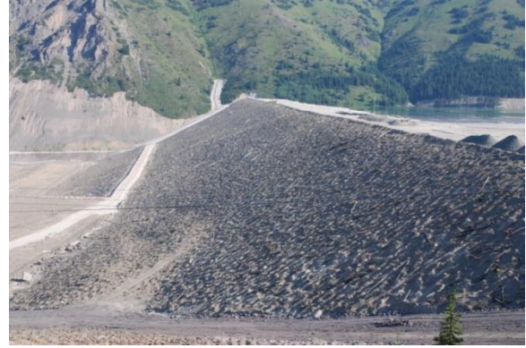
Photograph 1 (left) and 2 (right). Rough and loose surface configurations can be made using an excavator on slopes up to 2:1 or 26°. Large areas can be treated for a cost of about $700/ha.
