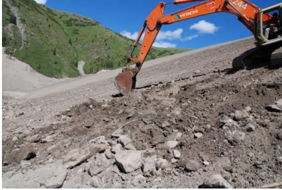
Photograph 1 (left) and 2 (right). Rough and loose surface configurations can be made using an excavator on slopes up to 2:1 or 26°. Large areas can be treated for a cost of about $700/ha.
