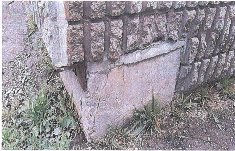
Photo 063 South-West Corner Foundation
