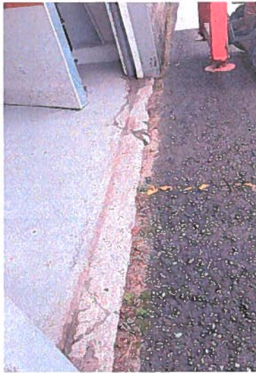
Photo 018 Apron Slab Under Garage Door
