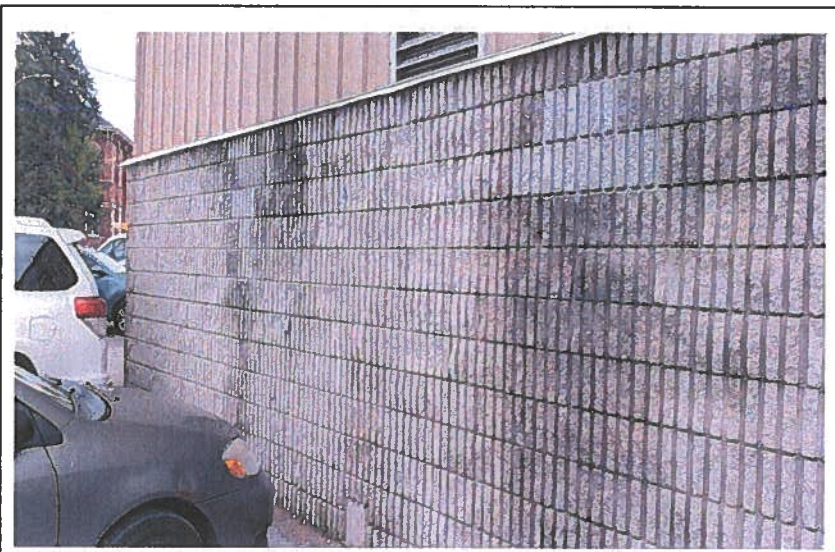
Photo 068 Architectural Precast Concrete Wall Panels
