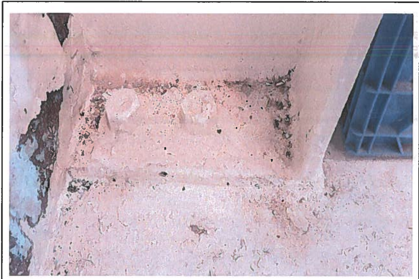
Photo 007 Pre-Eng Frame Base Connections
