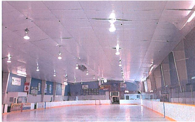
Photo 002 Roof Deck Insulation covering Pre-Engineered Frames
