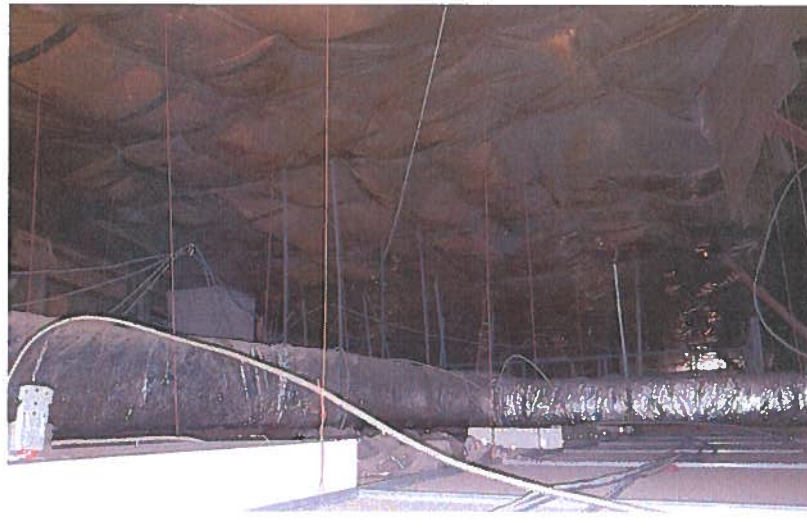
Photo 058 Insulation and Plastic Covering
