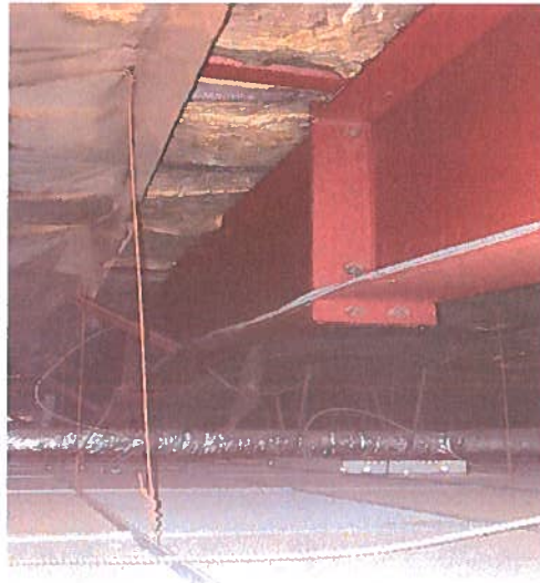
Photo 057 Partial Second-Floor Roof Framing
