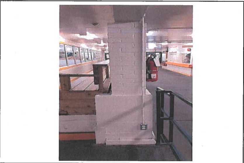
Photo 044 Columns in Lobby
