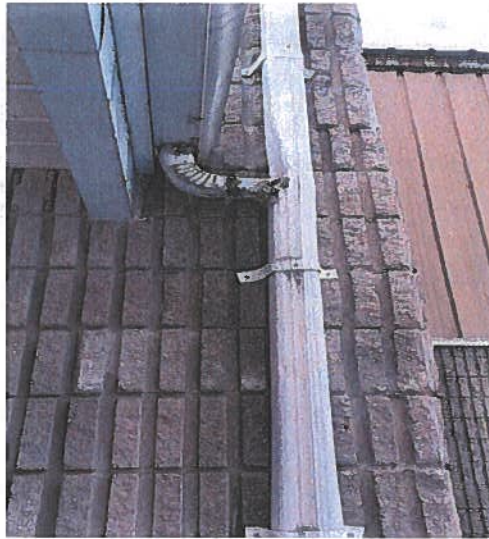
Photo 072 Damaged Eaves
